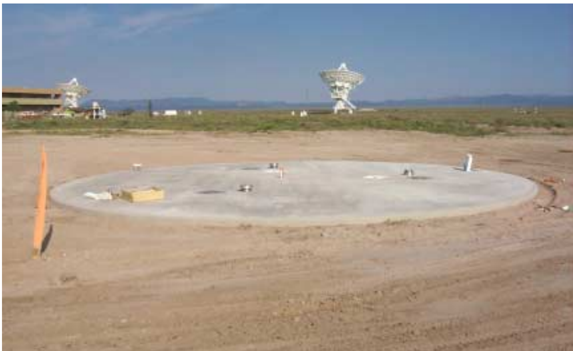
Figure 4.1.2. Completed foundation for VertexRSI antenna at the VLA site.
